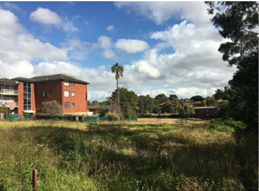
1. VIEW FROM CROYDON ST
